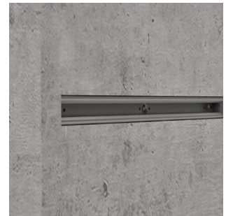
4.) No left overs should be within the channel slot. Any residue should be scrapped out
