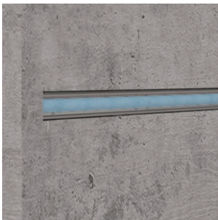
1.) After pouring of cement, the concrete wall should be left to dry
