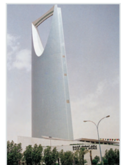
Kingdom Centre, Riyadh
