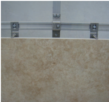
Sub channel support system provides adjustable in lateral direction. This enables quick positioning of the anchors along the horizontal channels to meet the T31 bolts fixed on the back of the stone panels.
