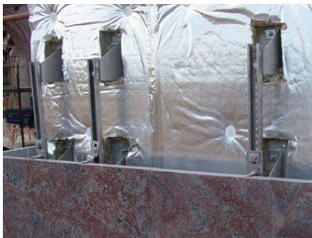
Sub channel support system designed to bear heavy loads at projection sizes exceeding 40 cm. Stone panels are installed using T31 undercut bolts.
