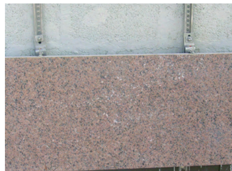
A flexible and rigid sub channel system suitable to take the variation in projection sizes and turn in corners. T31 and suitable anchors accommodate this system to enable secure installation.
