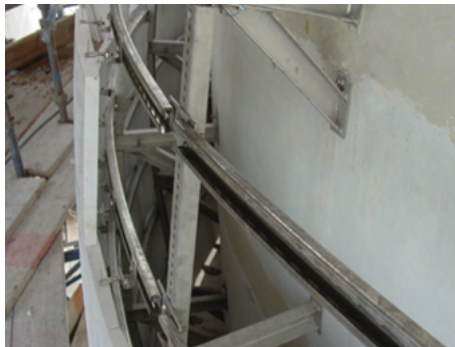
Sub channel support system provides adjustable in lateral direction. This enables quick positioning of the anchors along the horizontal channels to meet the T31 bolts fixed on the back of the stone panels.
