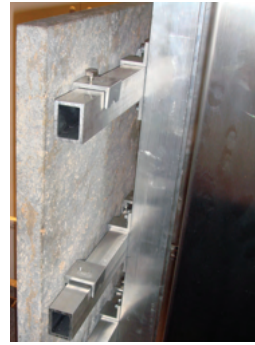
Sub channel support system provides adjustable in lateral direction. This enables quick positioning of the anchors along the horizontal channels to meet the T31 bolts fixed on the back of the stone panels.
