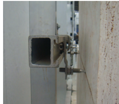
A flexible and rigid sub channel system suitable to take the variation in projection sizes and turn in corners. T31 and suitable anchors accommodate this system to enable secure installation.
