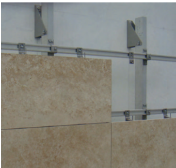
Sub channel support system designed to bear heavy loads at projection sizes exceeding 40 cm. Stone panels are installed using T31 undercut bolts.
