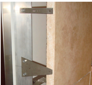
A flexible and rigid sub channel system suitable to take the variation in projection sizes and turn in corners. T31 and suitable anchors accommodate this system to enable secure installation.
