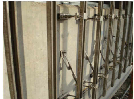
A flexible and rigid sub channel system suitable to take the variation in projection sizes and turn in corners. T31 and suitable anchors accommodate this system to enable secure installation.
