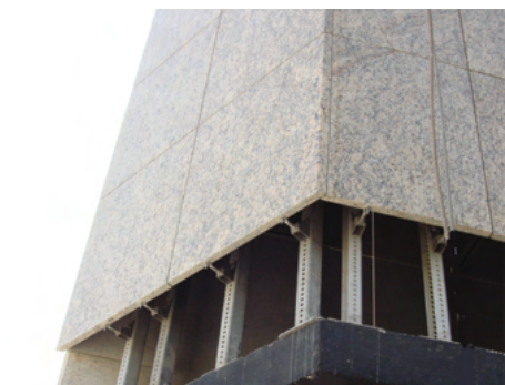
Sub channel support system provides adjustable in lateral direction. This enables quick positioning of the anchors along the horizontal channels to meet the T31 bolts fixed on the back of the stone panels.
